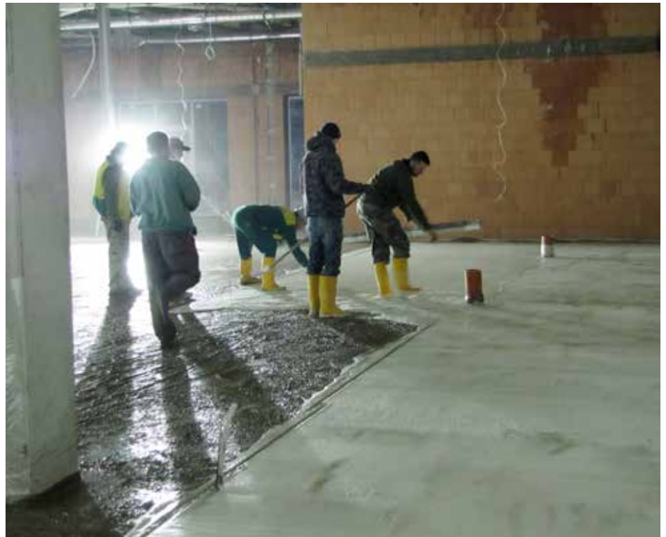
Sikafloor®-3+ CorCrete application in the building materials merchant Dek Znojmo outlet in Czech Republics. Refurbishment of 1200 m 2 concrete slab with the color Light Grey.
