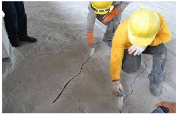
Non-moving crack repair. Opened crack is filled and injected by using Sikadur®-52 or Sikafloor®-156 epoxy resin.
