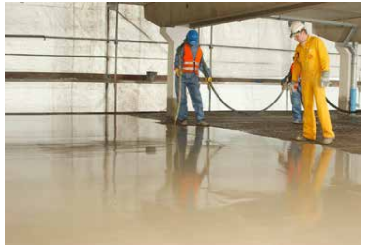
Application of Sikfloor®-30 Level overlay in a parking deck.
