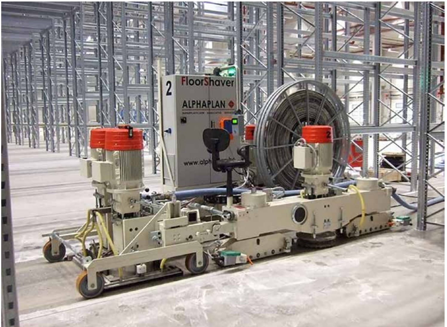
Fast and dust-free AlphaPlan FloorShaver grinding robot producing ultra-flat floor surface.
