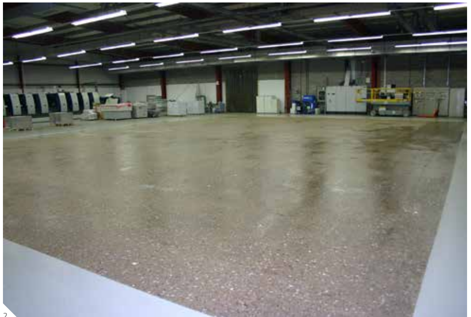
1 Strip installed concrete slab.
