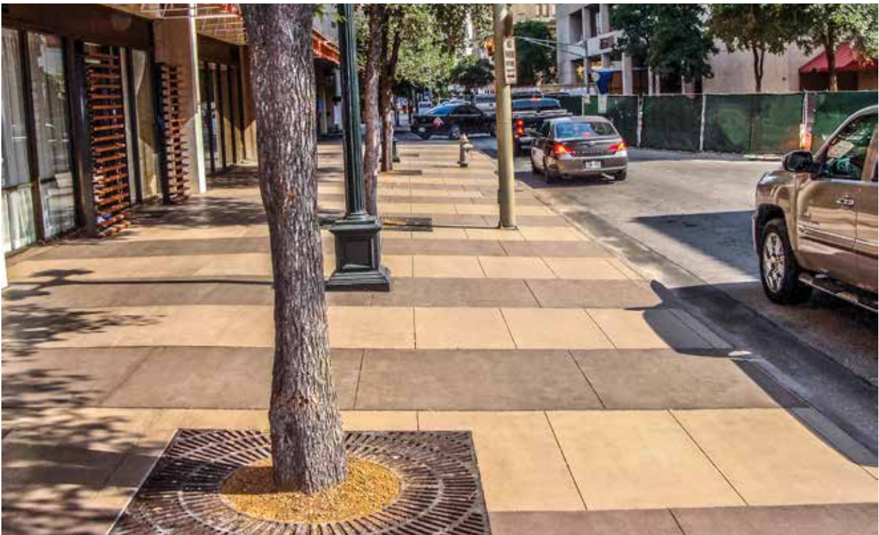
Integral colored pavement with Sika® concrete colorant.
