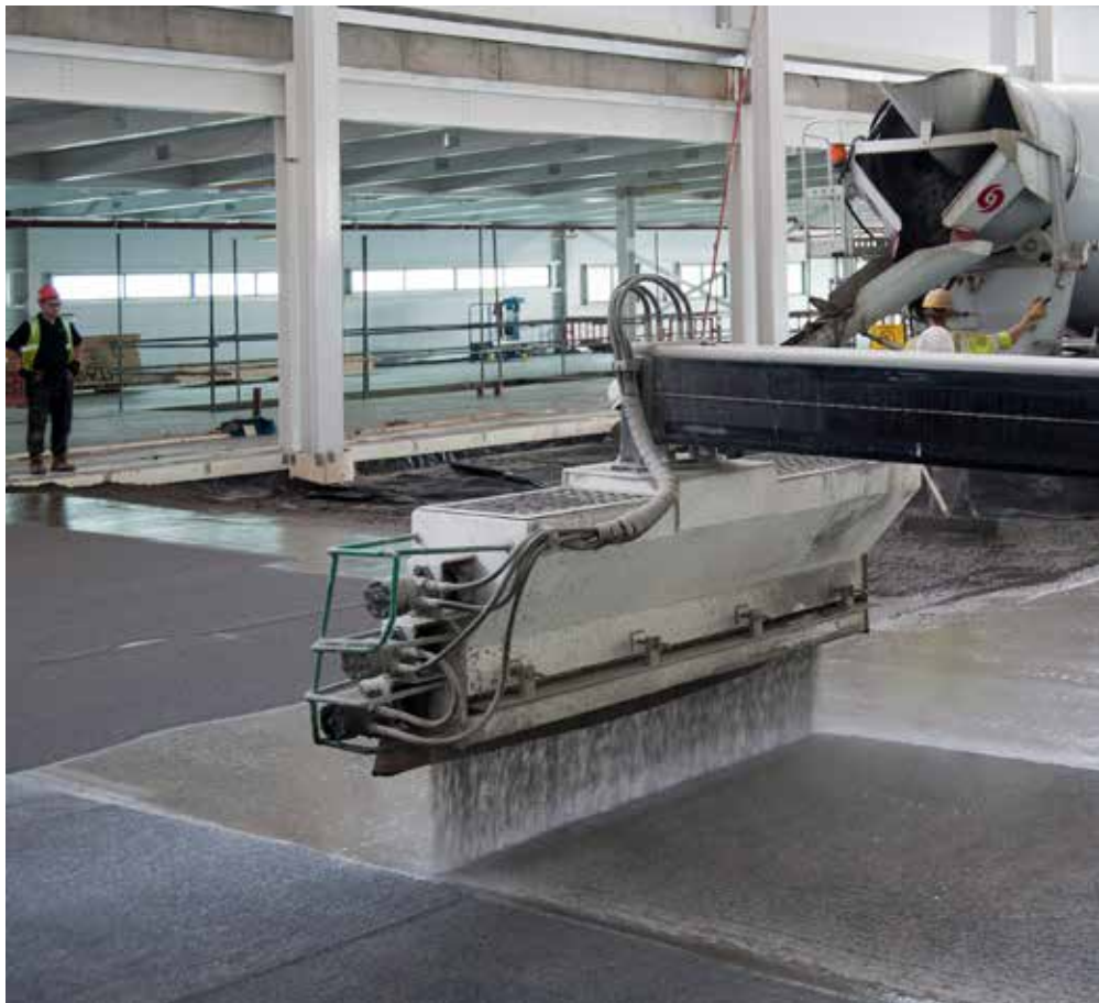
Mechanical spreading of Sikafloor®-2 SynTop dry shake hardener on fresh concrete.
