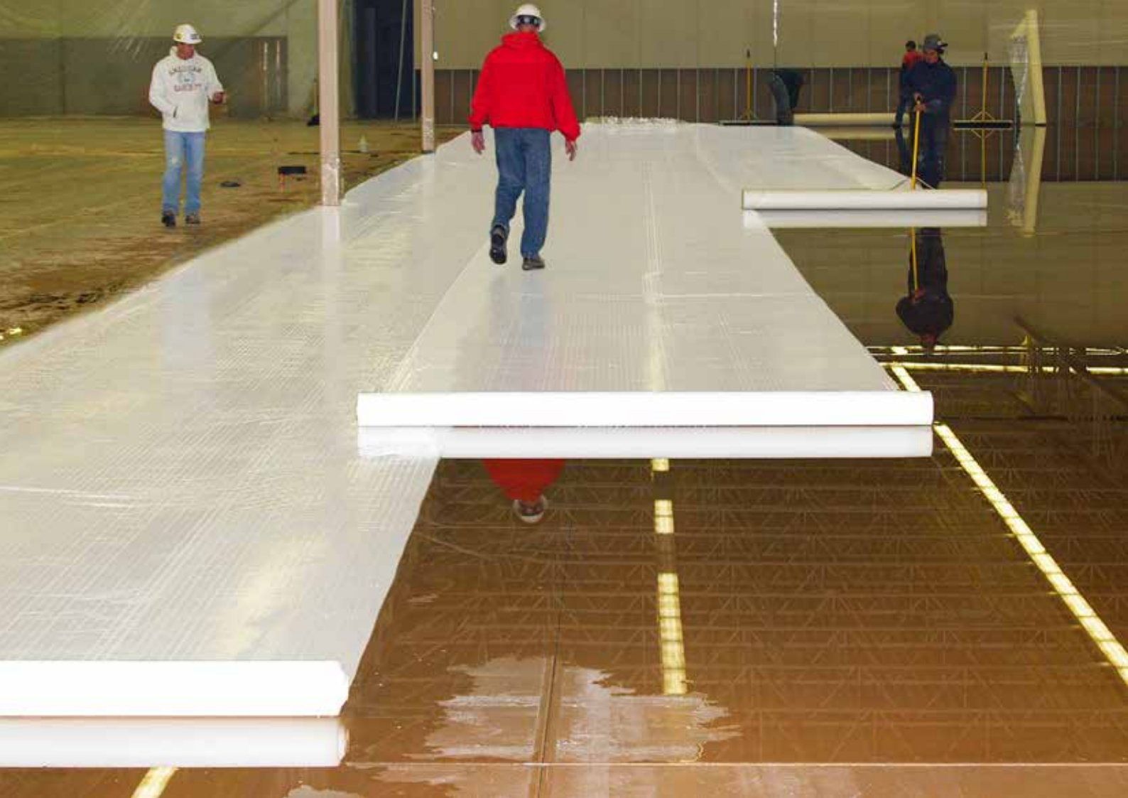
An ultimate curing solution: Sika® Ultracure water retaining blanket system combines wet and sheet curing methods.
