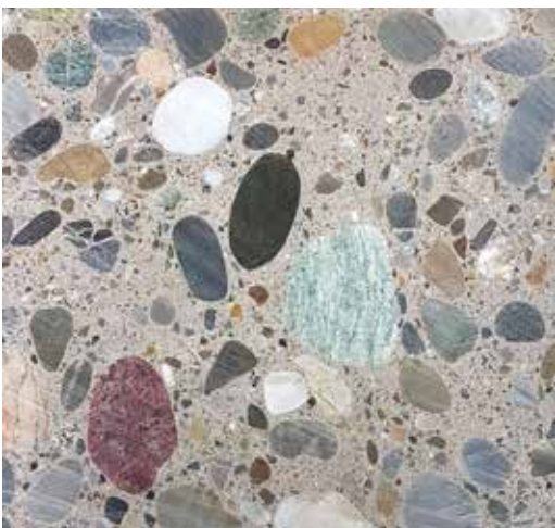
Cut section of hardened concrete.
