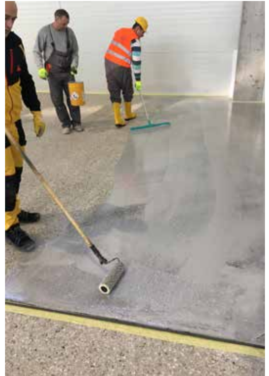
SikaScreed® HardTop repair screed system enables fast application. While in the back the team is still placing the screed, in the front the power floating can start in 90 minutes.
