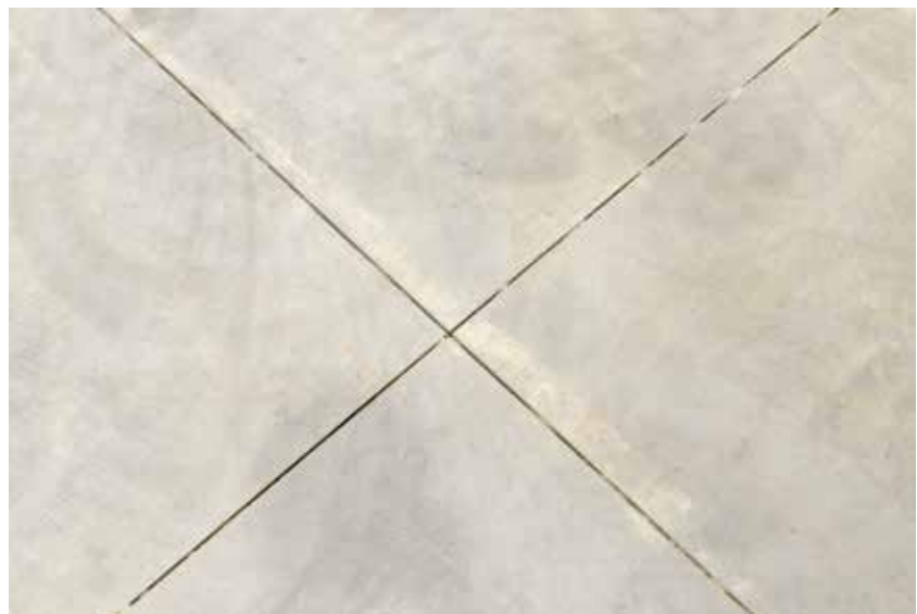
Saw-cut contraction joints accommodate the initial shrinkage of the concrete slab.
