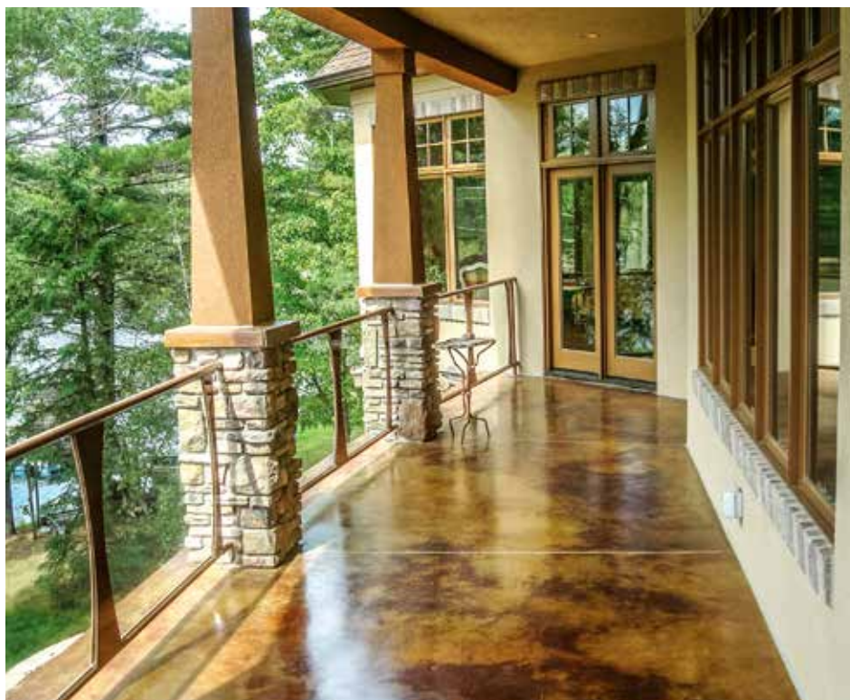
With Butterfield Color® reactive acid stains colored external concrete slab.
