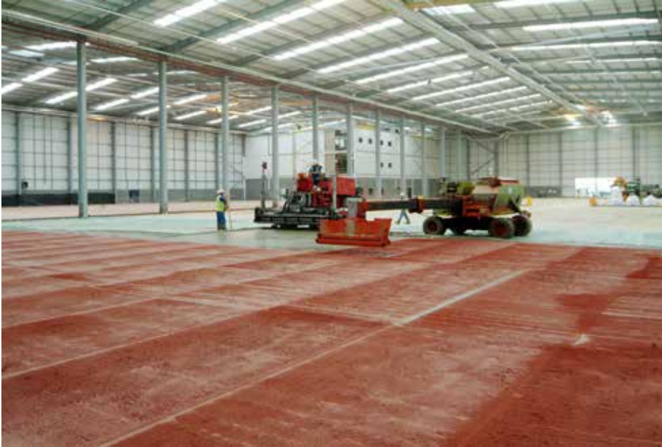
Colored Sikafloor®-3 QuartzTop application.
