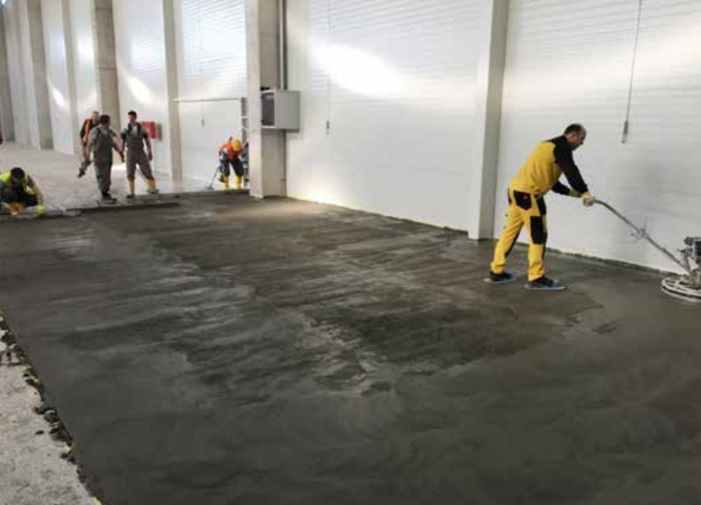
SikaScreed® HardTop repair screed system enables fast application. While in the back the team is still placing the screed, in the front the power floating can start in 90 minutes.
