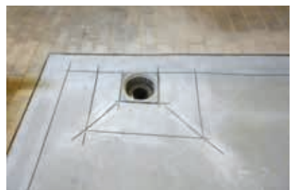
SATURDAY MORNING: Substrate preparation after curing of the screed.
